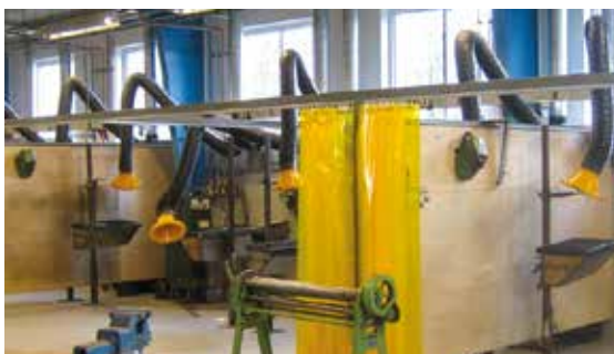
Wing arms ø160mm 3m installed at technical school. Including automatic control devices for automatic start/stop of fan and motor damper.
